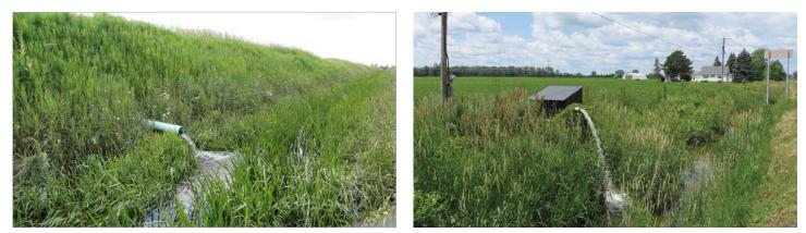
Figure 6. (a)(left) Subsurface drainage outlet flowing into a drainage ditch, and (b)(right) a nearly level field with not enough grade to allow gravity flow of the drainage water into a shallow drainage ditch, so the drainage water flows into a sump from which it is pumped out to the ditch.
