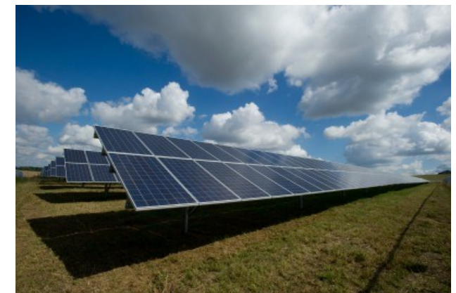
Utility grade solar projects are being sited throughout Michigan.
