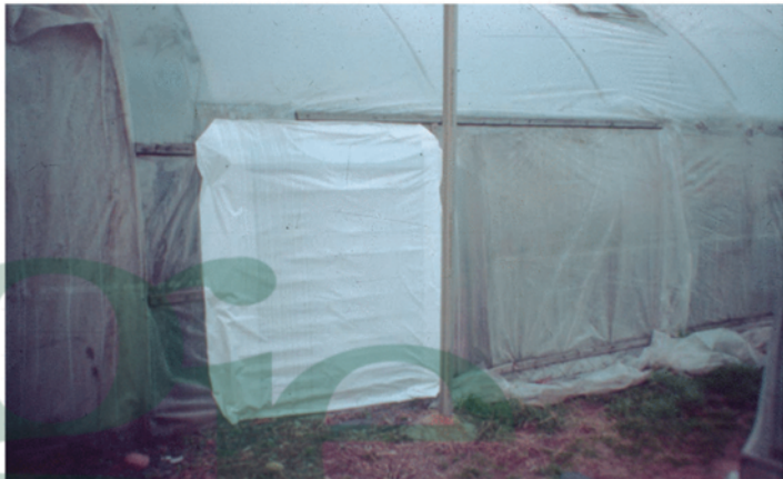
A simple method of reducing heat loss is to cover the shutter or fan with a layer of plastic film
