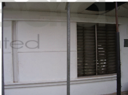
A more permanent solution to reducing heat loss is to install a piece of 1-inch thick insulation board and attach it over the fan shutter.
