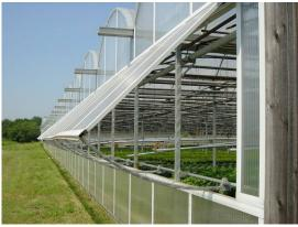
**Picture 1.** Fully opened side wall ventilation window in a mechanically ventilated greenhouse.
