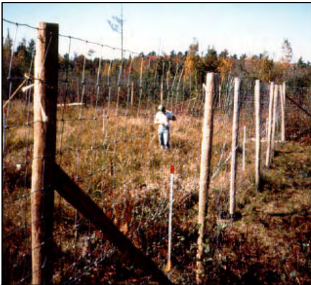
An 8'-tall woven wire fence is effective but expensive (UPTIC photo).
